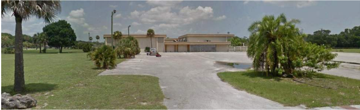
Facing north toward property from Brentwood Drive
