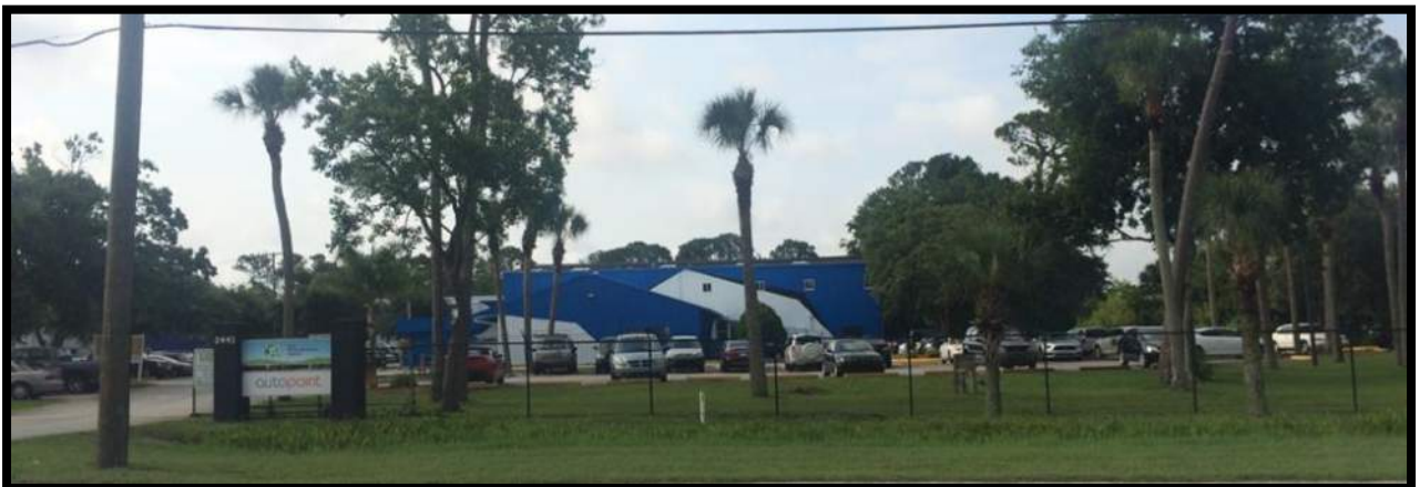
Drainage Ditch along Bellevue Avenue
