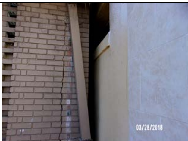
View showing separation between subject and 730 E. ISB building. Note cracking of wall.
