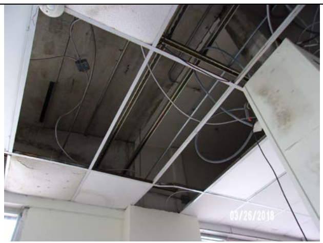
Additional missing roof tiles. Note appearance of mold on column
