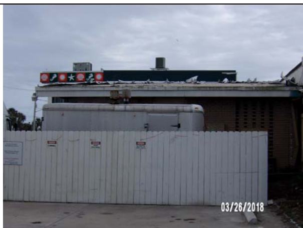
Facing south showing groundwater remediation unit. Note peeled back roof panels on subject building
