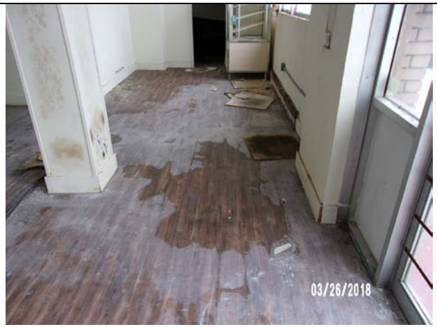
Pooled water evidencing roof leaks
