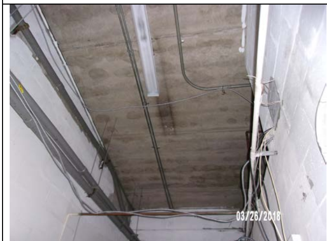
Missing ceiling tiles revealing poured concrete roof slab
