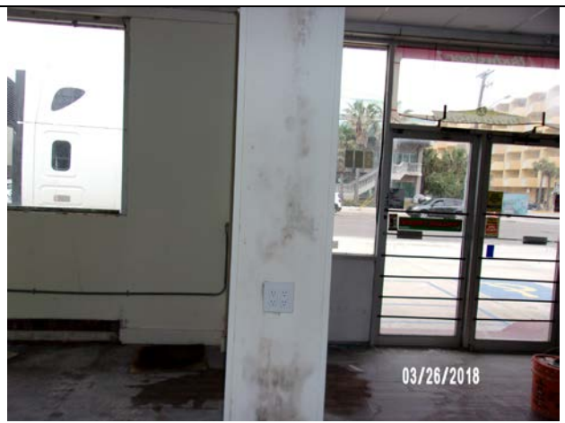
Additional indications of likely mold (on column)
