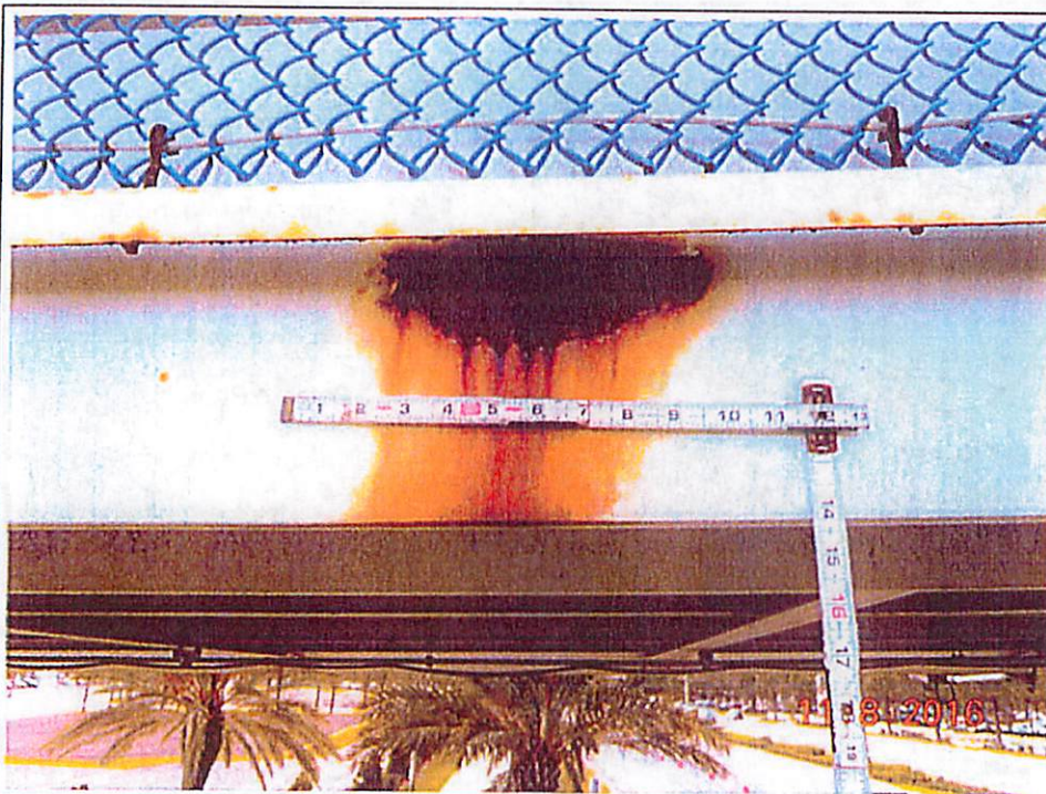
UNIT 0 Photo 8 120 Steel Truss
