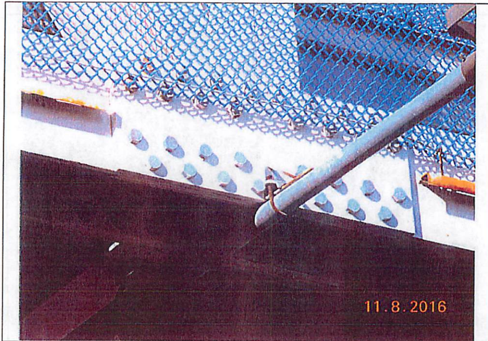
Typical Bolted Splice (Bottom Chord shown)
