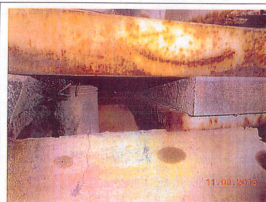
UNIT 0 Photo 4 310 Elastomeric Bearing
