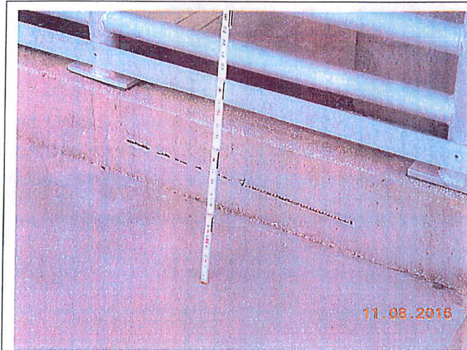
UNIT 1 Photo 25 8099 PS Conc Slab (Sonovoid)
