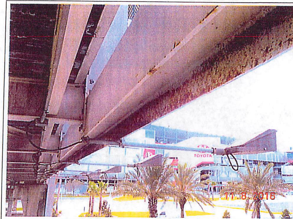
UNIT 0 Photo 7 120 Steel Truss
