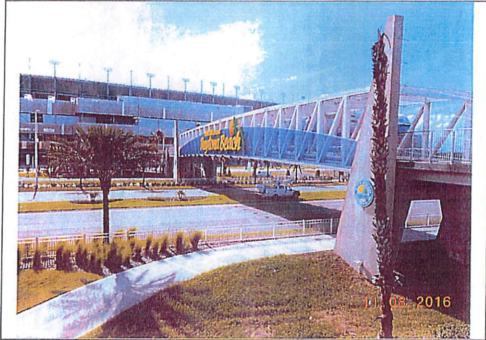
Outside Elevation of Truss
