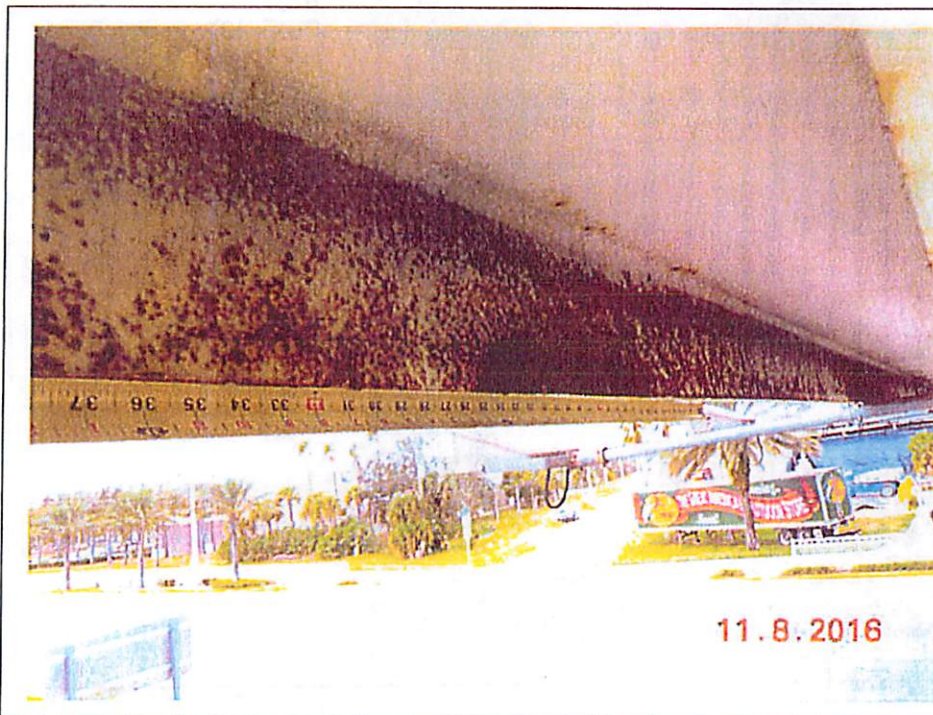
UNIT 0 Photo 10 120 Steel Truss
