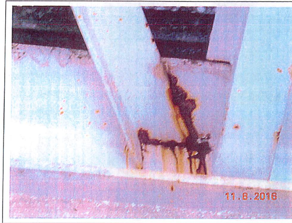
UNIT 0 Photo 21 152 Steel Floor Beam
