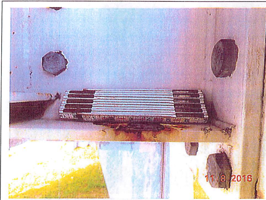
UNIT 0 Photo 22 152 Steel Floor Beam
